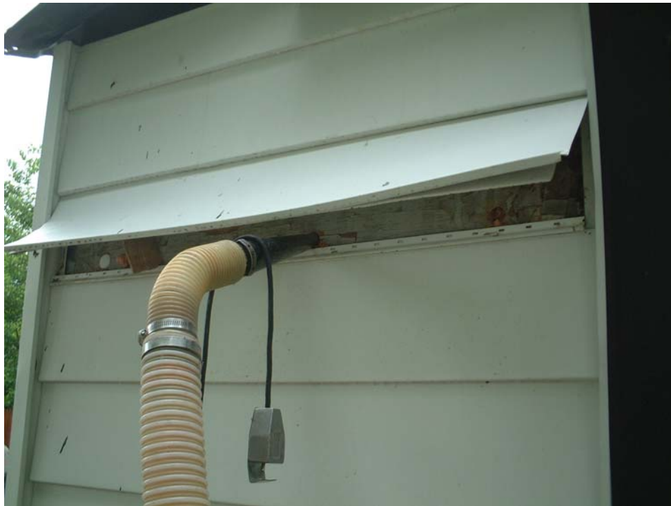
Installation of Blown-in Insulation
